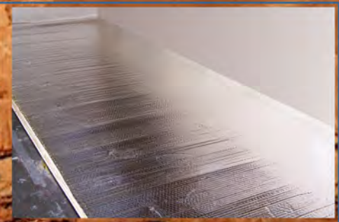
Reflective Insulation Blanket Applied to Roof, Slide-Out Floor, Entire Underbelly, Additional Wrap Around Holding Tanks
