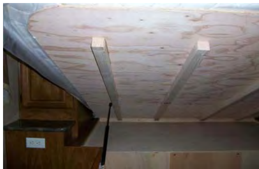
Plywood Under Bed
