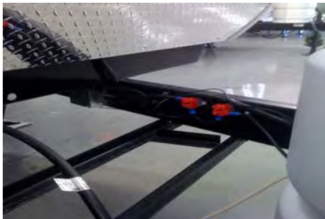
Not Off Road Frame Exposed Wiring
