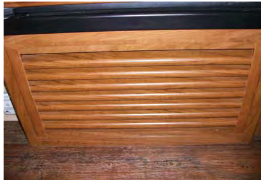
Custom Built Wood Return Air Vent
