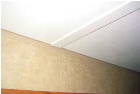
Stapled On Bat Moldings Fall Down Over Time
