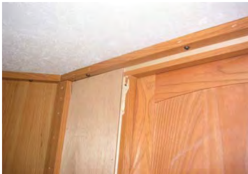
Stapled Together Cabinetry Throw Away Construction
