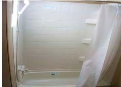
Residential Style Shower Walls
