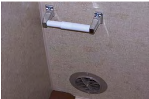
Ducted Heat into Bathroom
